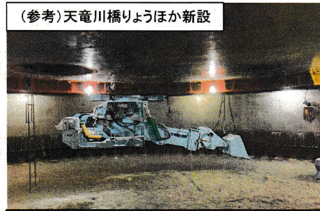
④掘削・沈設
